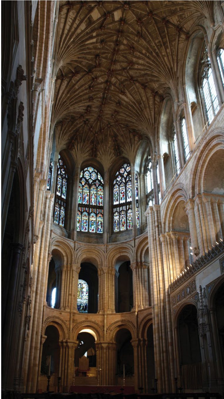
Figure 1: The presbytery of Norwich Cathedral. Although the current clerestory was remodelled in the 15th century, the disjuncture between Romanesque and gothic architecture above the first floor is a direct result of damage caused on St Maur(us)'s Day 1362. (Photograph by the author).
